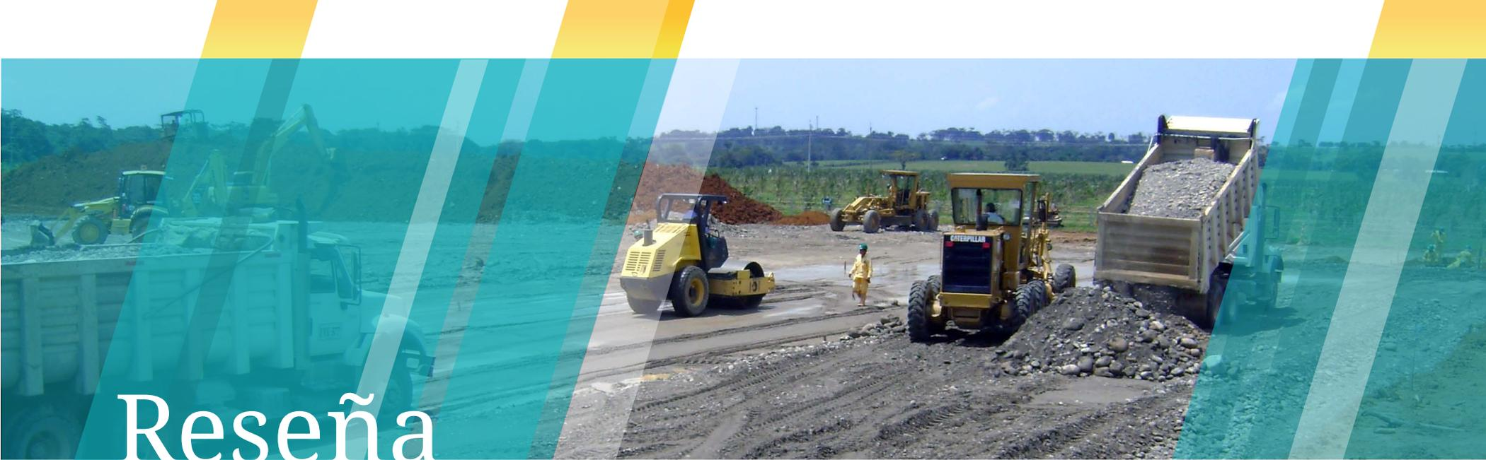
A wide-angle photograph of a construction site. In the foreground, a yellow Caterpillar roller is compacting a gravel surface. To its right, a yellow Caterpillar wheel loader is parked near a large pile of gravel. In the background, a white dump truck is dumping its load. A worker in a yellow safety vest is visible near the roller. The scene is set in an open field with trees and a clear sky in the distance. The image is overlaid with a semi-transparent teal and yellow geometric pattern.
